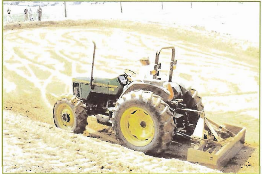
Figure 1 – The subgrade must be smooth, firmly compacted, and be free of water-collecting hollows.
