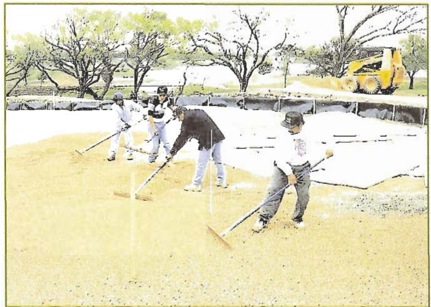
Figure 3 – Gravel drainage blanket installed to proper depth by using grade stakes.
